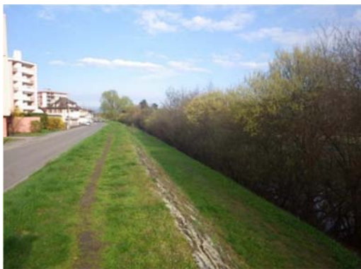
Figure 5. Illustration of the good reconciliation of the GEMA and PI issues. a bank protected by plant techniques and a dike kept in grass favoring the diversity of environments.
